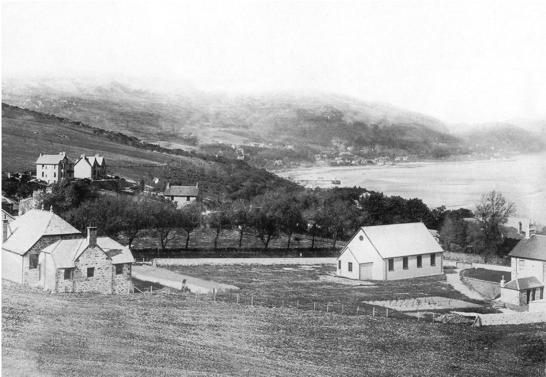
Believed to date between 1912 and 1919, and to have been taken from the top of the golf course, this picture shows the original tin Kames Free Presbyterian church (centre right) with the manse (right). The later church building was constructed further up the slope, gable to gable with the original.*
